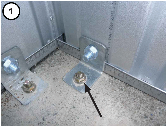
Inside view of typical anchor.
