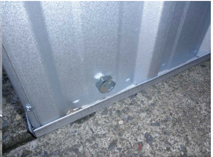
Outside view of typical anchor
