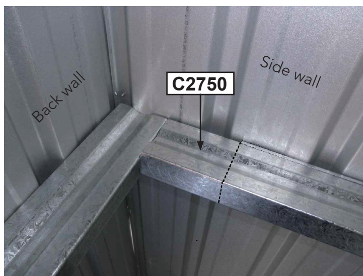
Previously installed wall bracing on the left and new gable wall bracing on the right.
